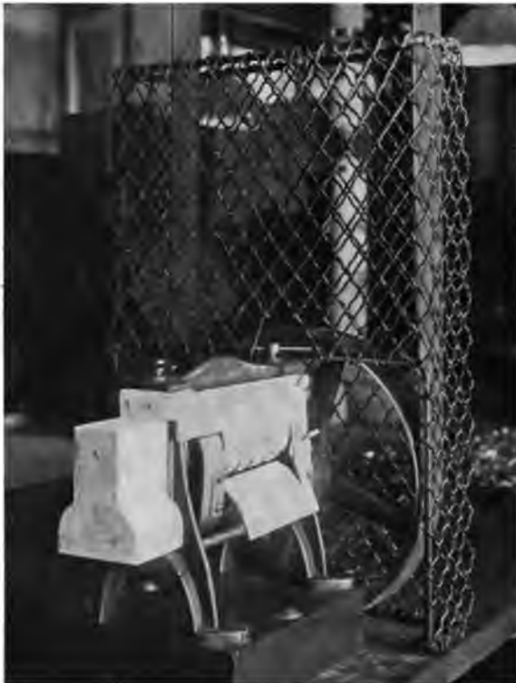
Fig. 3. Strap Creasing Machine with Guarded Rolls, Gearing, etc.*
